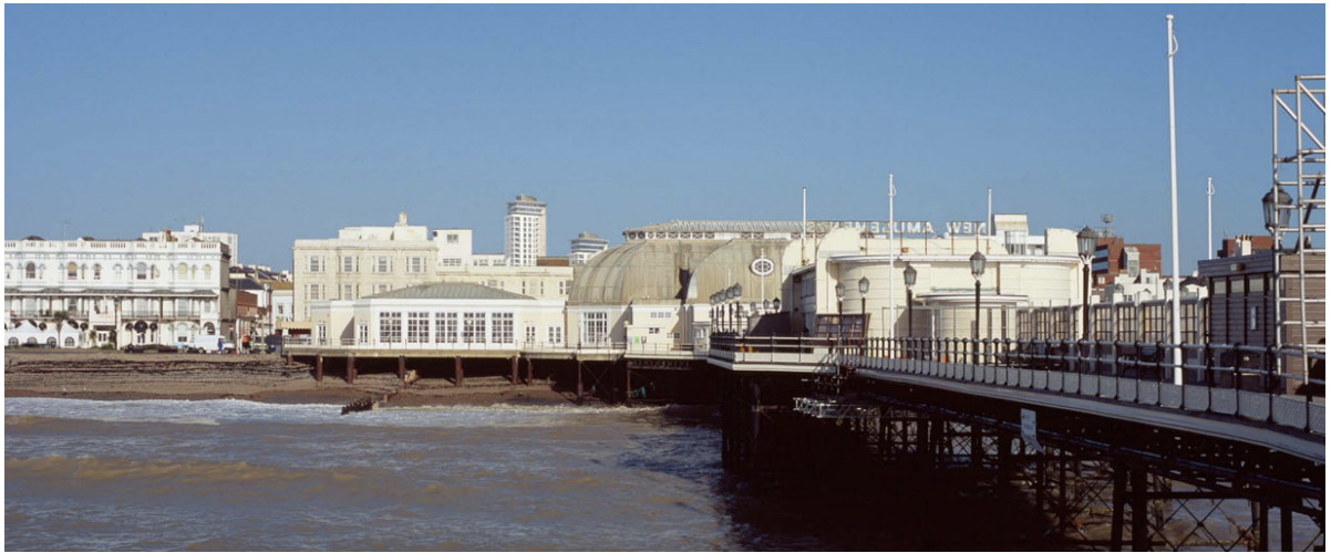
Looking North from the Pier
